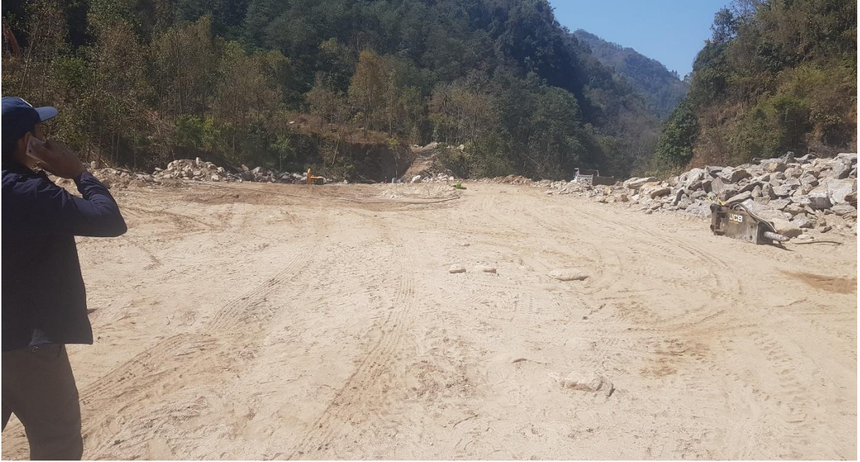
Figure 4: Earthwork in filling in desander area.
