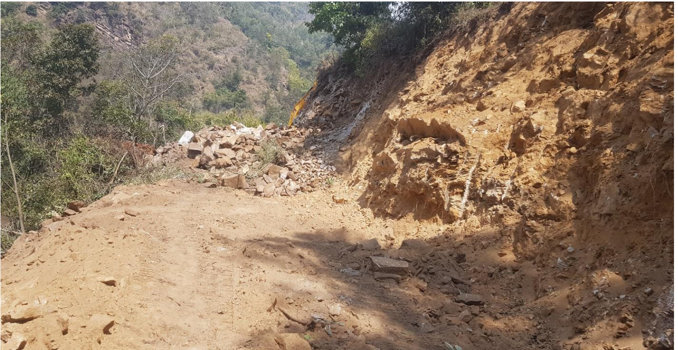
Figure 10: Road Widening for pipeline alignment.
