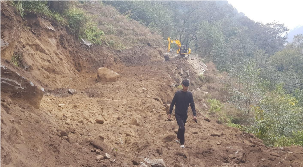
Figure 11: Road widening for Pipeline alignment.
