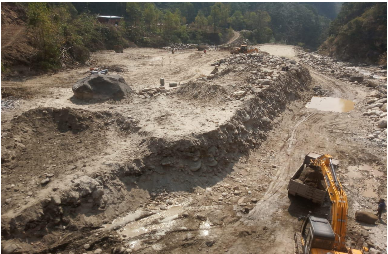
Figure 1: Excavation for headworks foundation.
