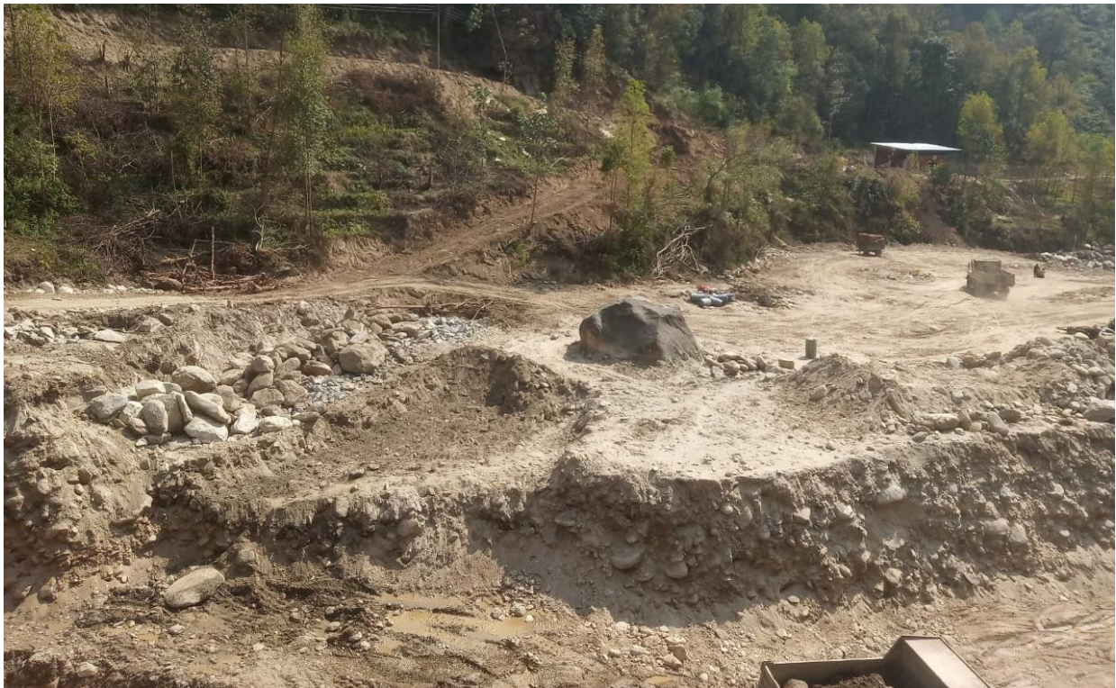
Figure 2:Excavation works in headworks area.
