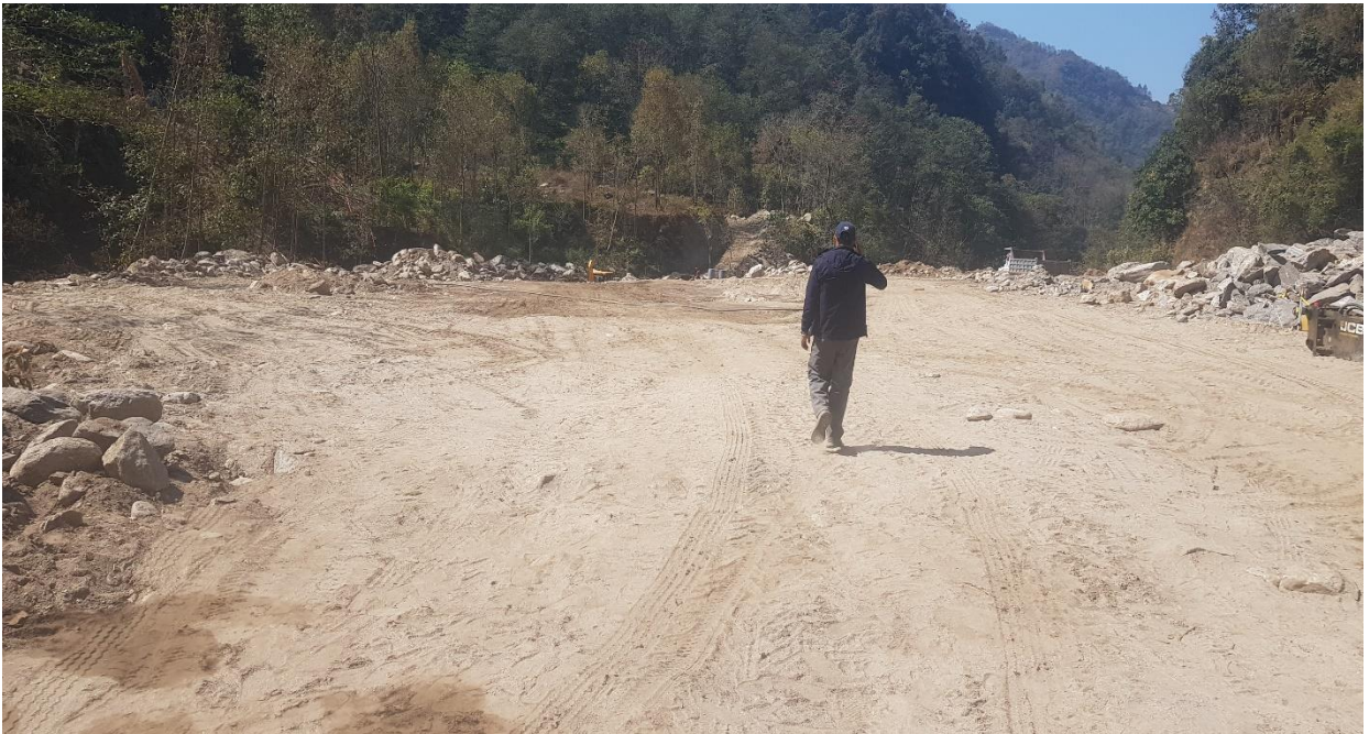
Figure 3: Earthwork in filling around desander area.
