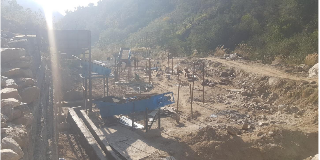
Figure 14: Crusher Plant installation works
