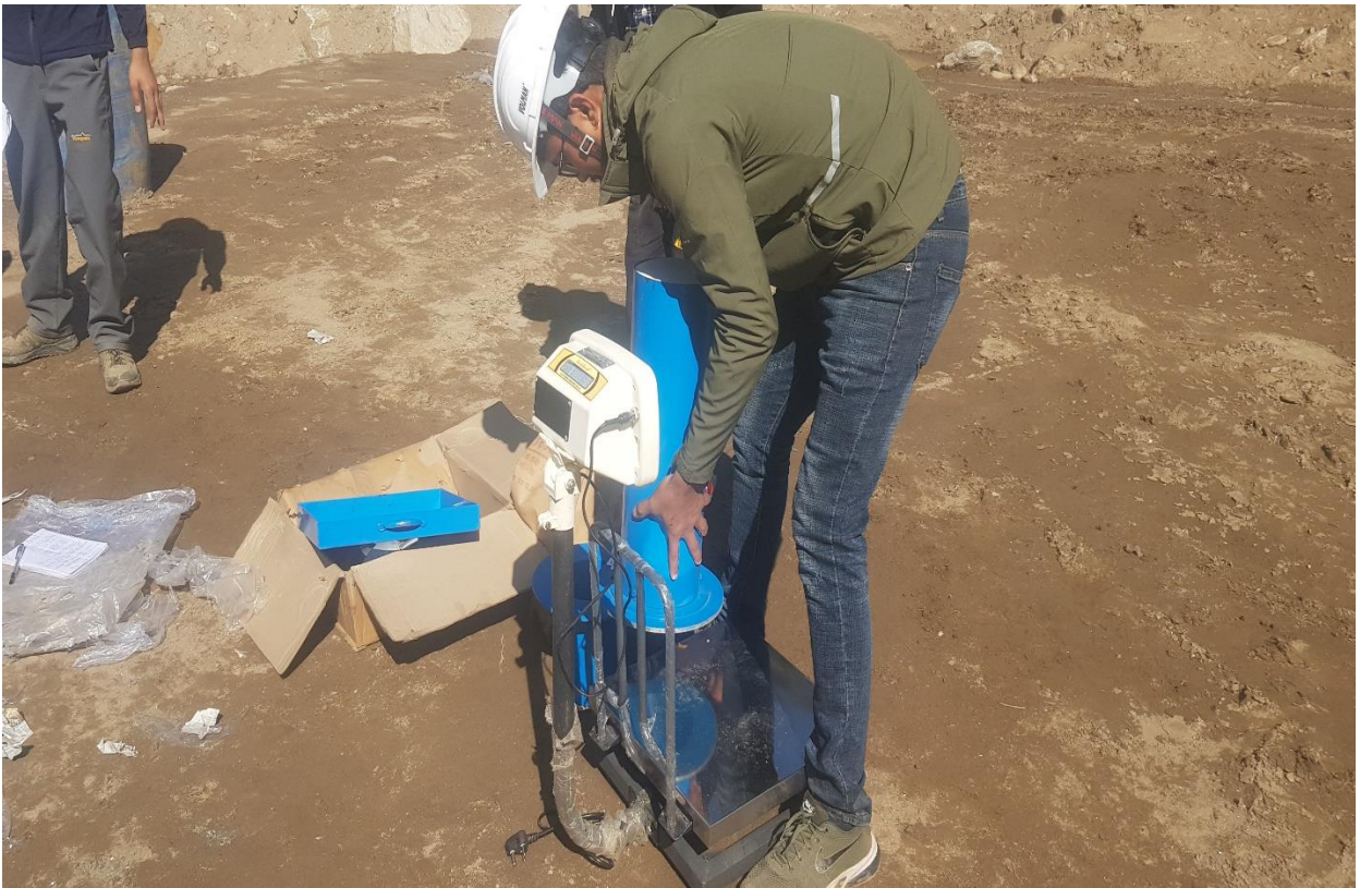
Figure 5: Compaction Testing In desander area.
