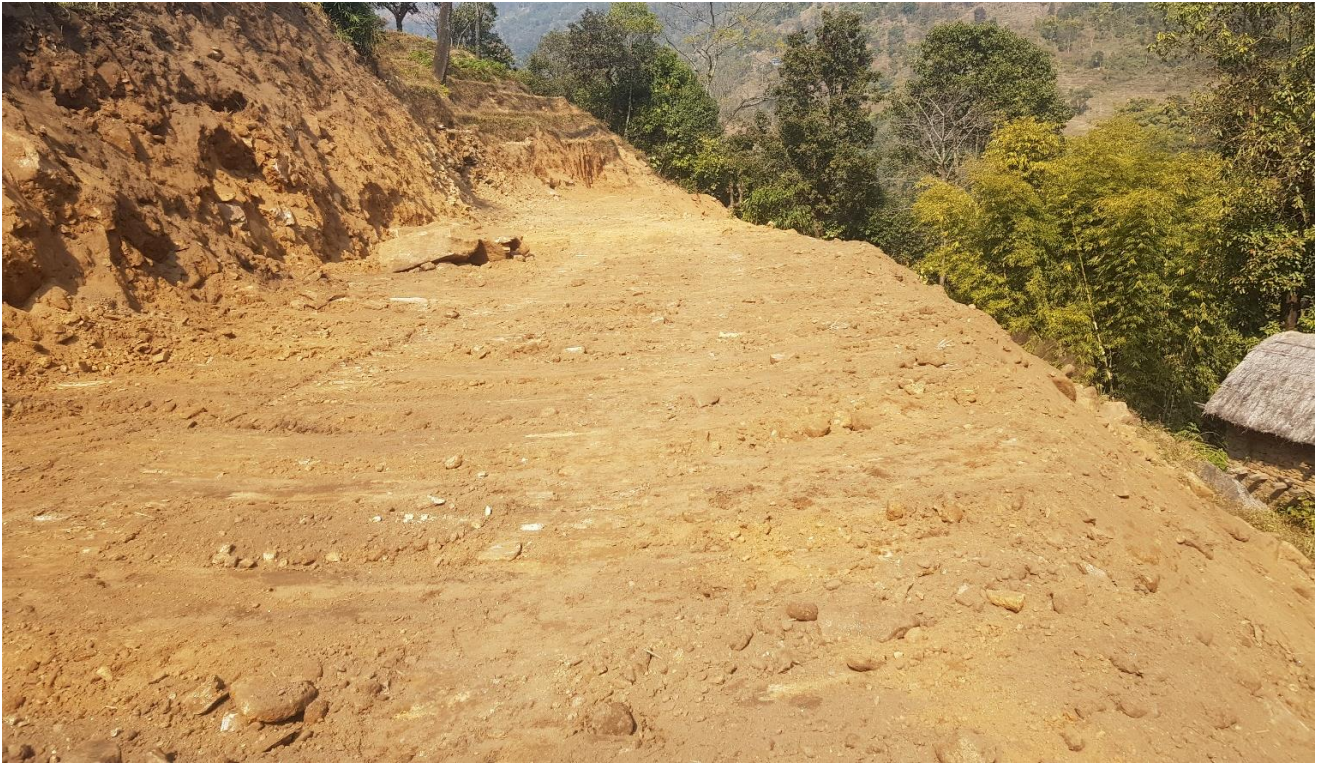
Figure 12: Road Widening for Headrace Pipeline Alignment
