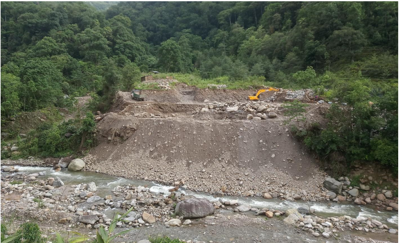
Figure 15: Excavation for Powerhouse Structures
