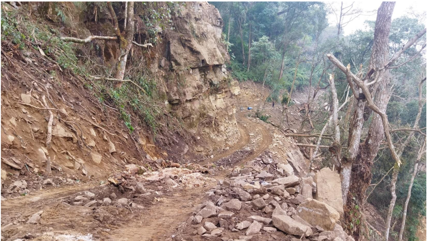
Figure 13: Construction of Project Road
