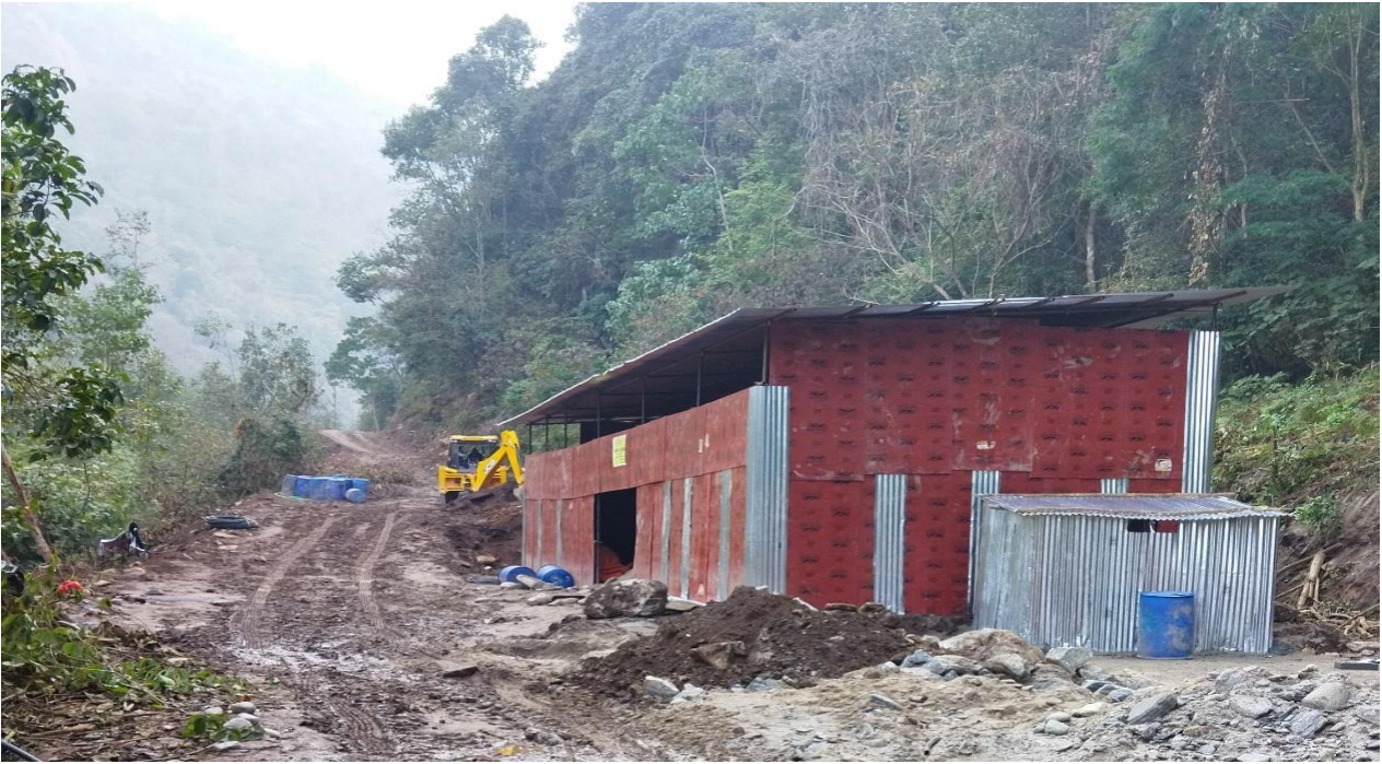
Figure 6: Labour camp at headworks
