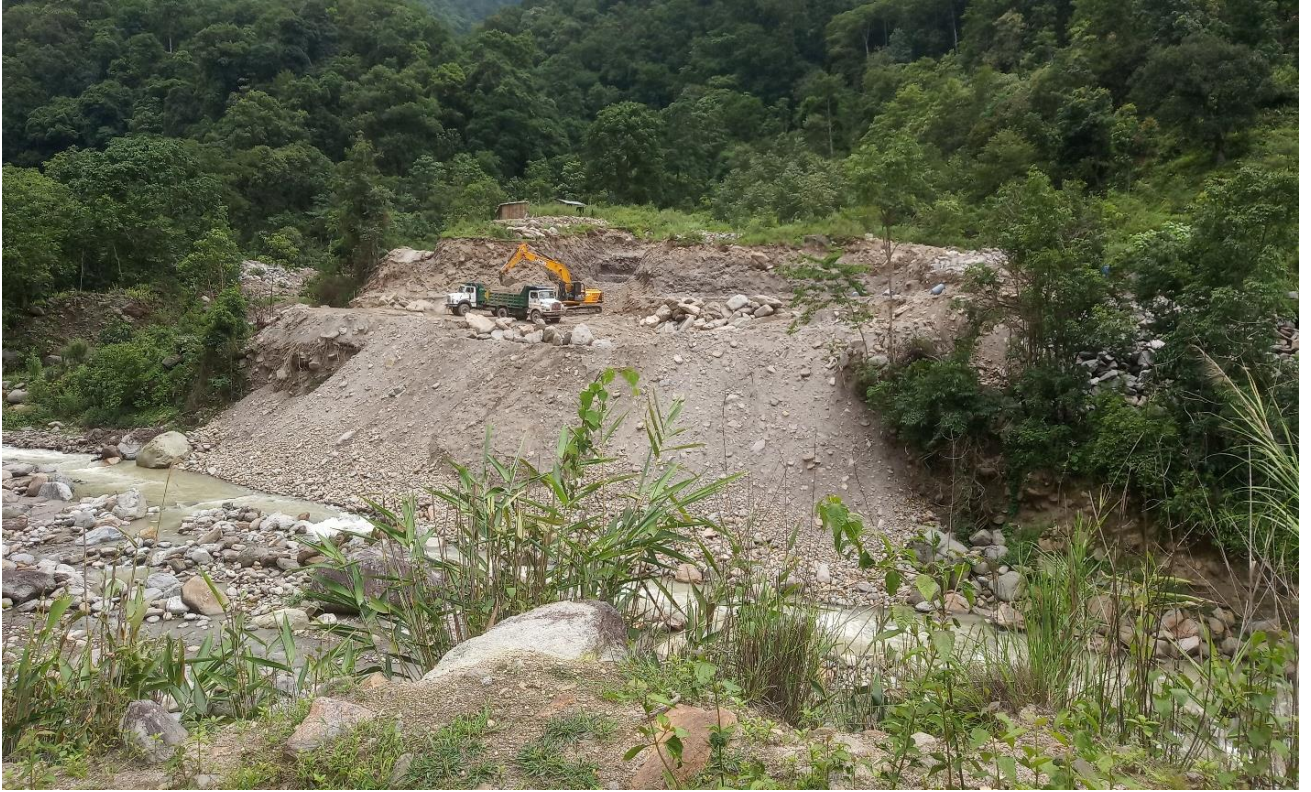
Figure 16: Excavation for Powerhouse Structures
